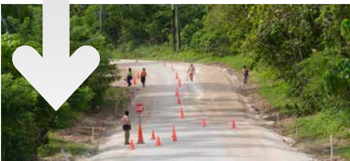
Base layer preparation for Momote-Lorengau road
