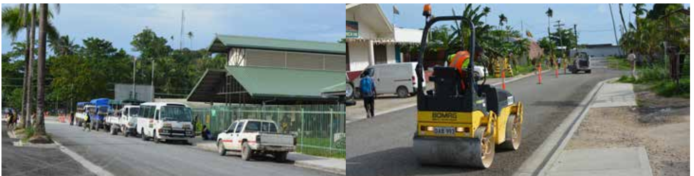
Road sealing around Lorengau Market
